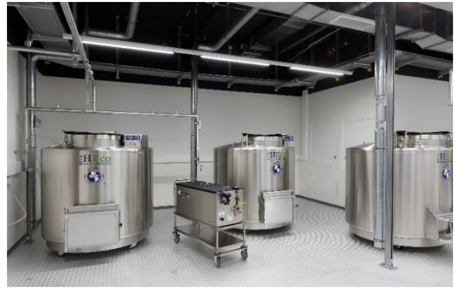
Manual storage in vapor phase of LN 2
